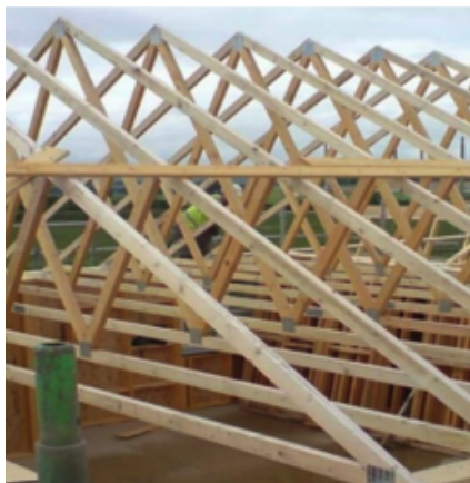
Figure 6: Framework of timber on the roof
